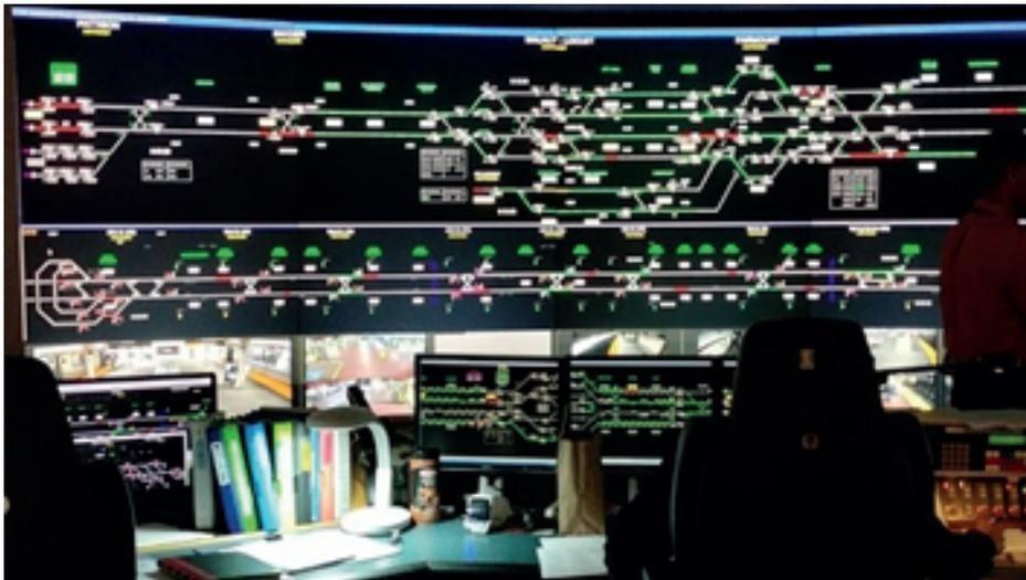
Fuente: T.Y. Lin International. (s.f.). MARTA's train control and SCADA system upgrade (TCSU) project. T.Y. Lin International, de <https://es.tylin.com/work/projects/martas-train-control-and-scada-system-upgrade-tcsu-project>
